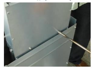
3. Slide the flue wrap over the flue
